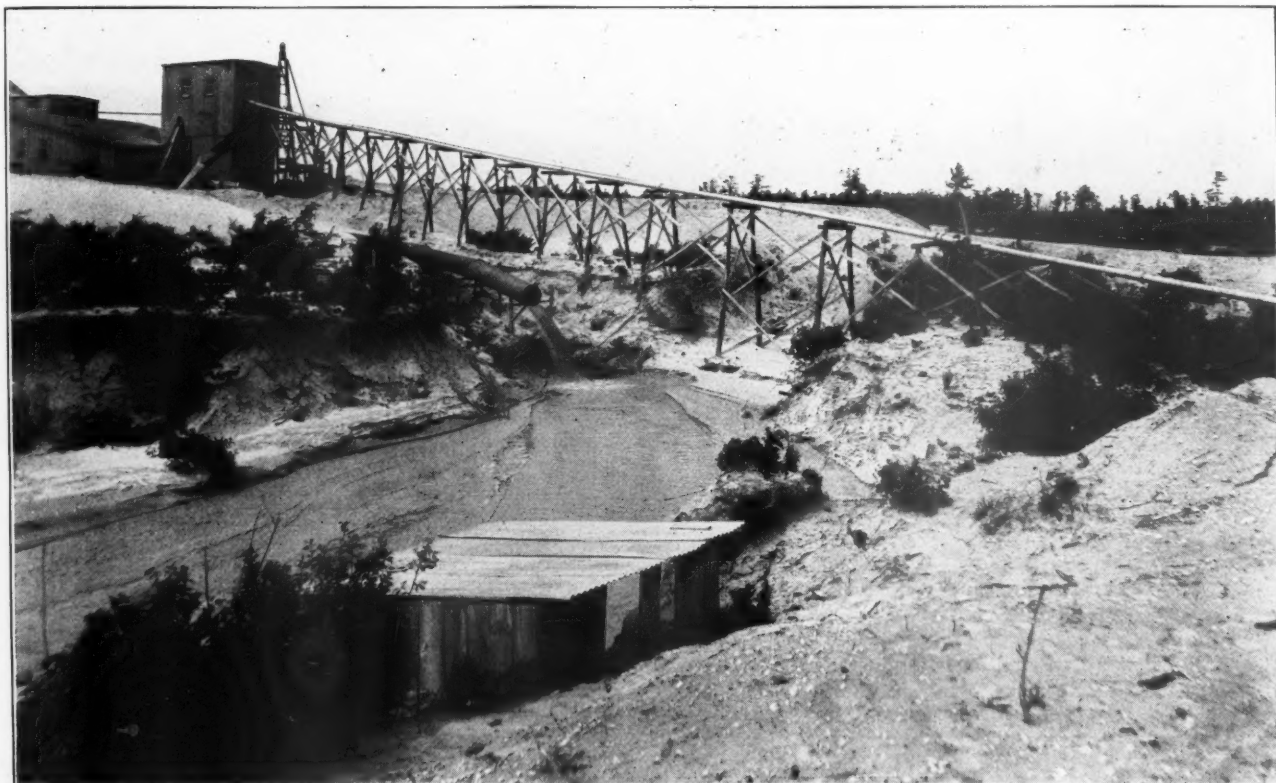
The Pump Line to the Plant and the Waste Pipe Discharging
